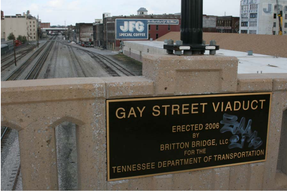
Figure 8: Northeast corner of site from the Gay Street Bridge; existing condition
