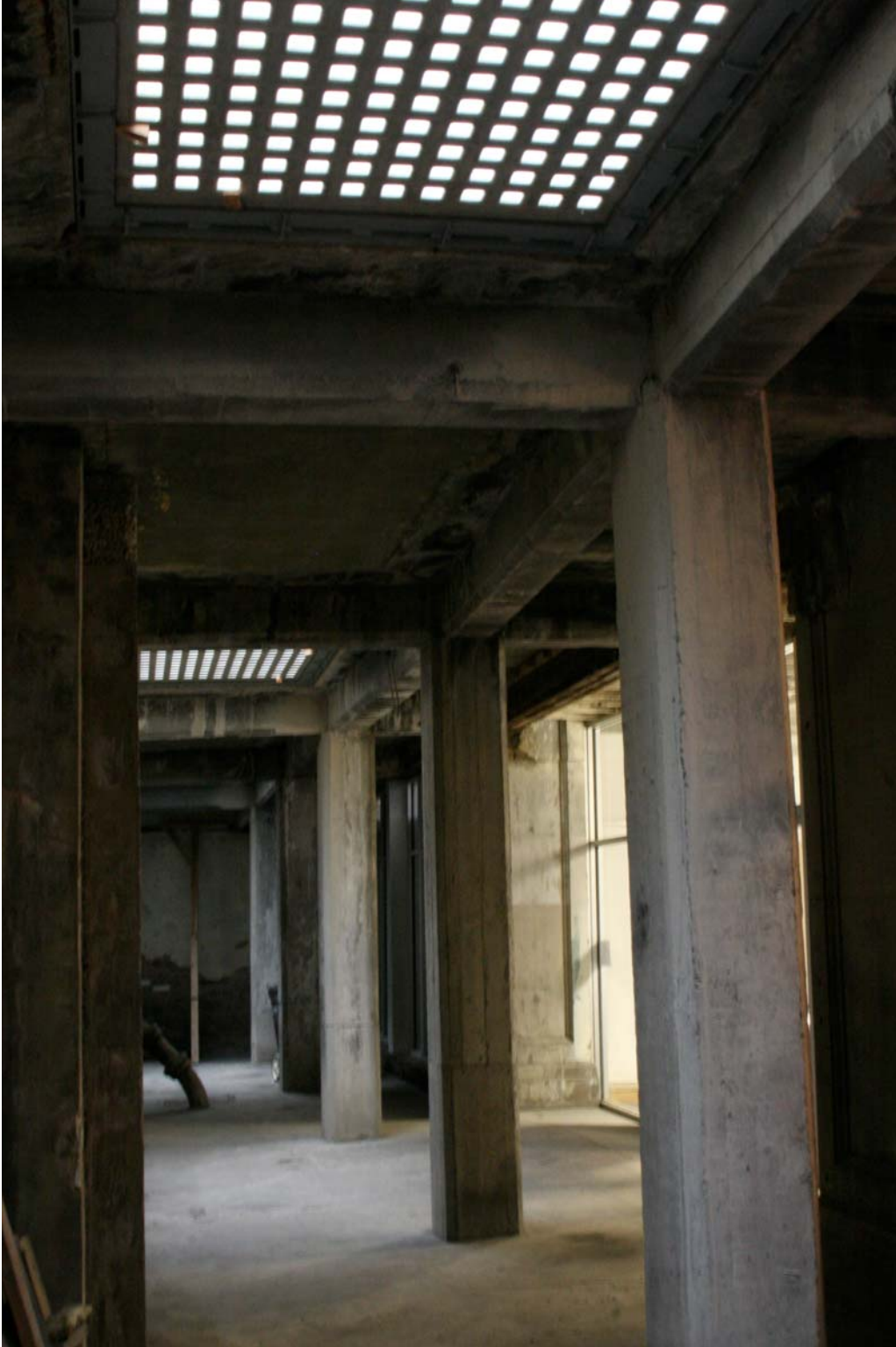
Figure 14: Underground Knoxville, showing glass tiles from sidewalk above. Image: Author
